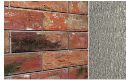
Joints between buildings
