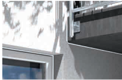
External connection joints
