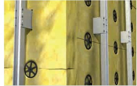
Insulating materials in rear-ventilated façades
